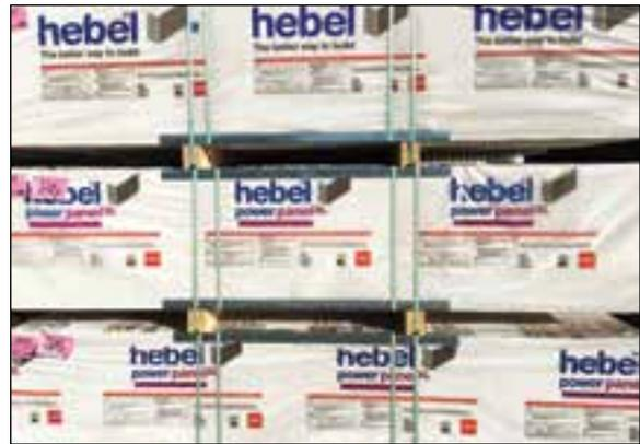
Figure 4.1.1 Stacking packs of Hebel PowerPanelXL
